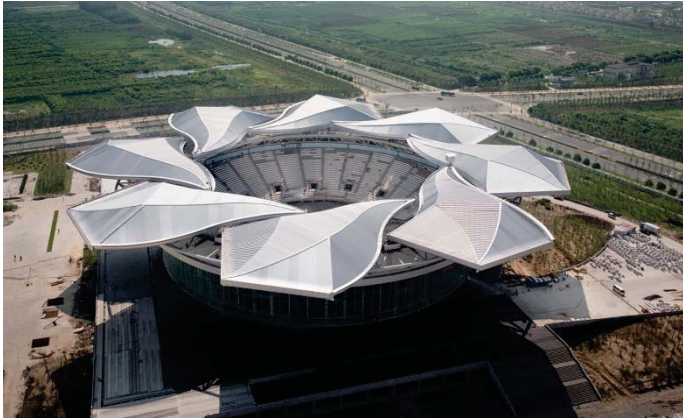
Figure 5. Qizhong Forest Sports City Arena - Roof open
