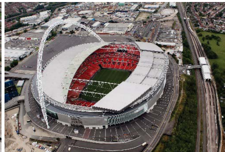
Figure 4. Wembley Stadium - Roof open
