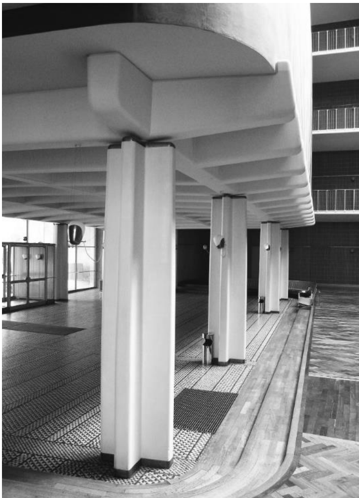
Figura 6: Column/Beam joint, Aarhus Town Hall, Arne Jacobsen Aarhus Denmark, 1941
