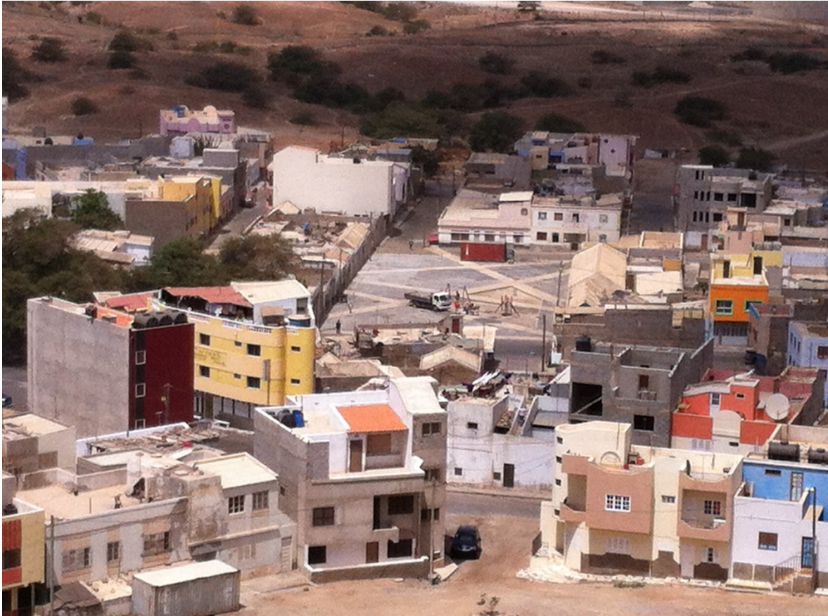
Figure 3: Houses in different stages of construction on Sal island, Cape Verde. © Kaian Lam
