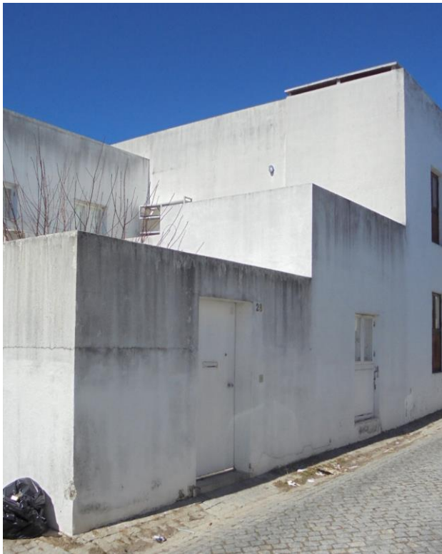
Figure 4: An example where the panel of the gate is white not creating contrasts in the façade.
