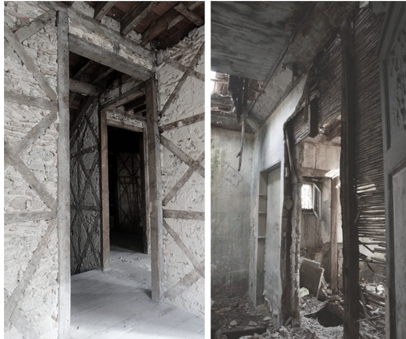
Figure 4: Internal timber frame wall: Pombalino building in Lisbon versus Bishop's Palace in Mileto (Calabria region) (2015, photo by author).
