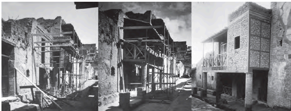
Figure 1: Reconstruction works of Casa a Graticcio (1929) [8]
