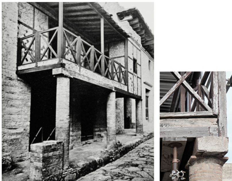
Figure 3: Casa a Graticcio (Insula III, 13-15, Herculaneum): main elevation after the 1930s restoration [16] and detail of L-shaped steel beams (2016, photo by the author).
