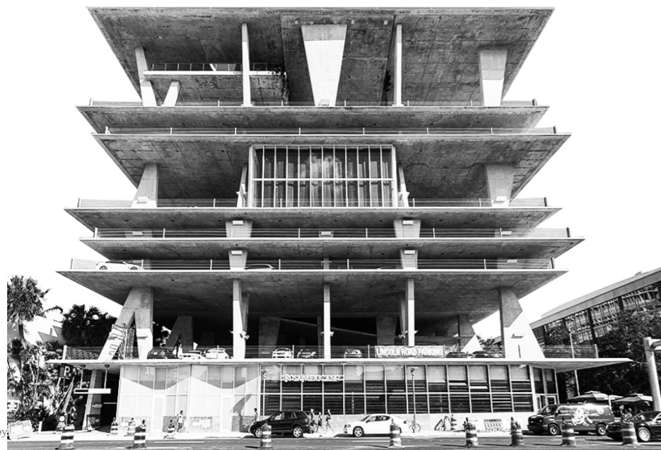
F09 1111 Lincoln Road Parking Garage by Herzog and de Meuron
