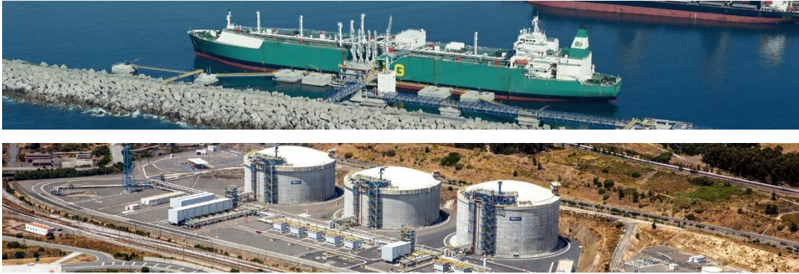
Figures 7 and 8: The TGN Terminal and the storage tanks
