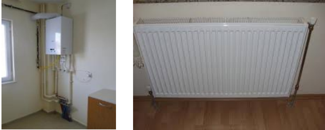
Figure 6: Gas fired boiler and radiator within dwelling
