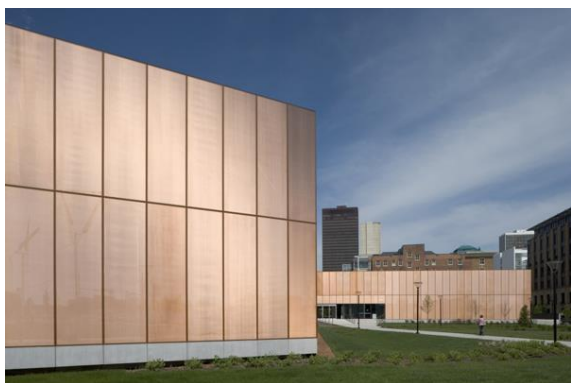
Biblioteca Publica Des Moines, David Chipperfield Architects, vidros com cobre expandido, Okalux
