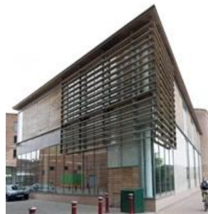
Piano Building, Garnett Netherwood – kidderminster, exemplo de pala horizontal fixa de madeira
