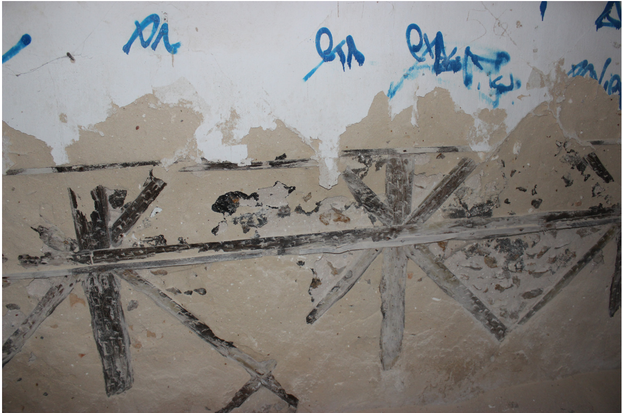
Parede interior no piso -1
