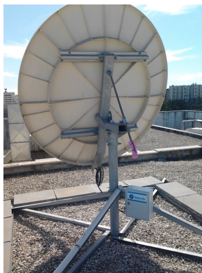
Figure 3.10: Parabolic dish and its support structure
