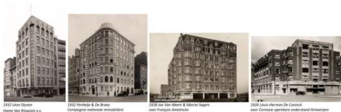
Figure 4. Amelinckx between prominent architects at the Jan Van Rijswijcklaan.
