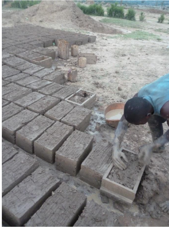
Building soil-bricks for houses
