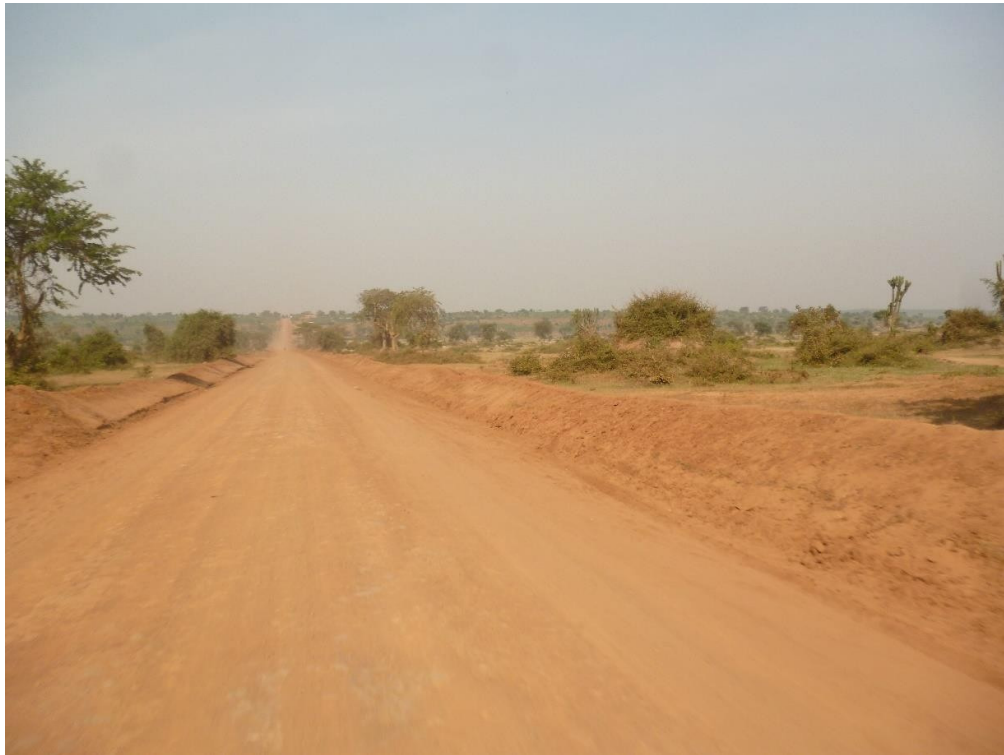
Road, which connects the Base Camp to Juru
